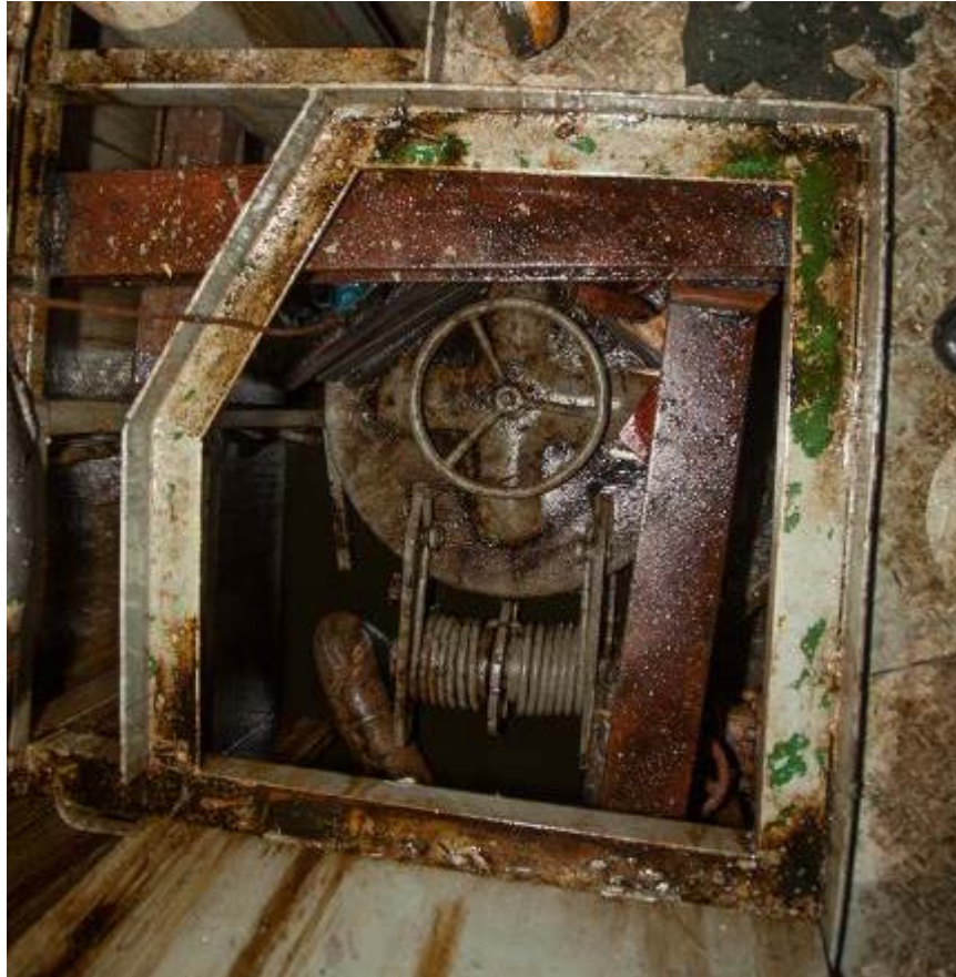
Figure 6 The hatch to the pipe tunnel
